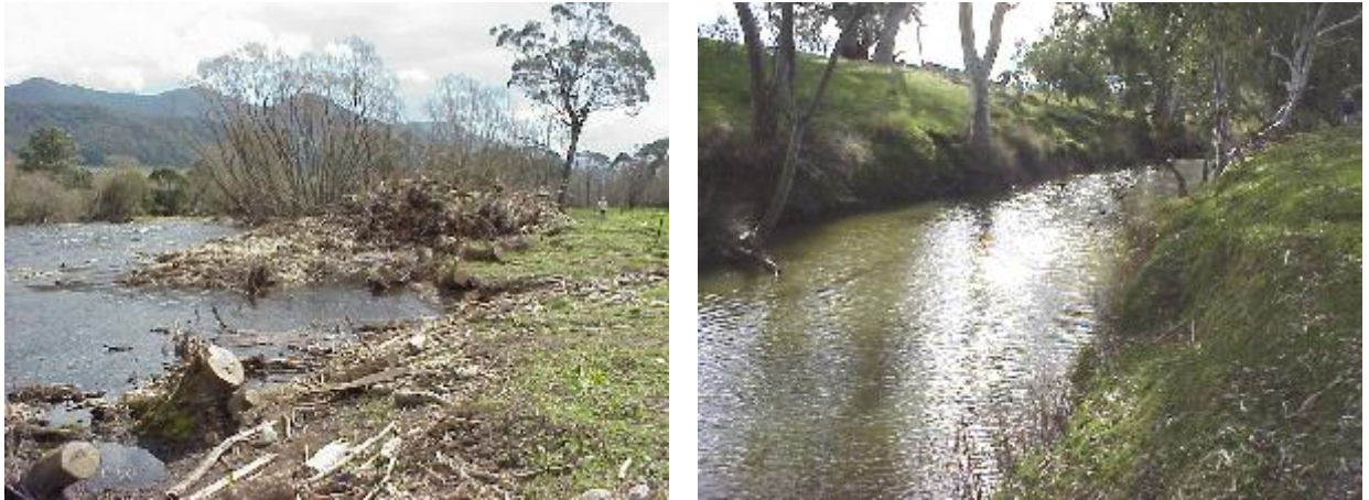
Figure 34 Kiewa River (left) from ‘alpine’ group and Bet Bet Creek (right) from ‘granite’ group both showing significant degradation in riparian zone.
